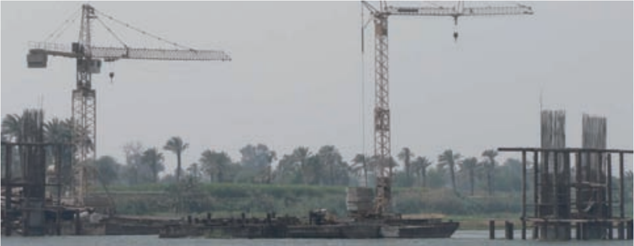
A new road bridge under construction across the Nile, linking the main west-bank highway south of Mallawi with the eastern desert near El-Bersheh. It is likely to offer direct road access to Amarna.
