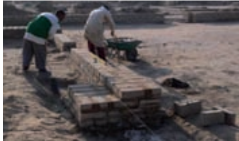
Local builder Mohammed Mahmoud Hussein at work, recreating the line of the front wall of the animal building.
